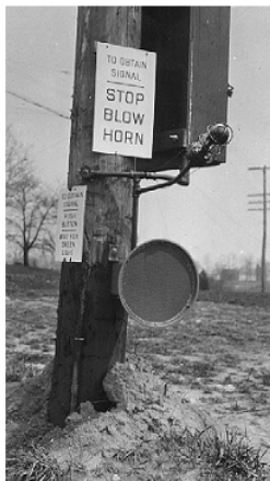
"To Obtain Signal - Stop Blow Horn," traffic-actuated signal light, Charles Adler, Jr. Collection, ca. 1920-1980
